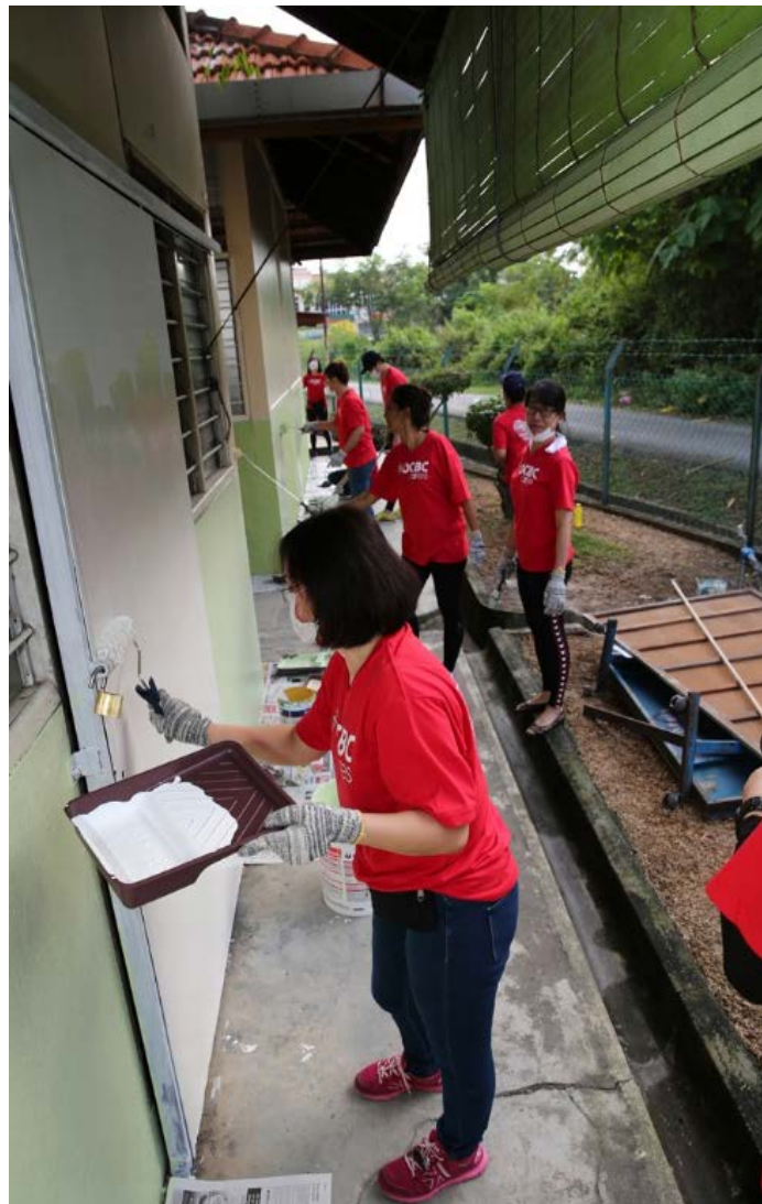
OCBC Bank staff volunteers painting the school walls
